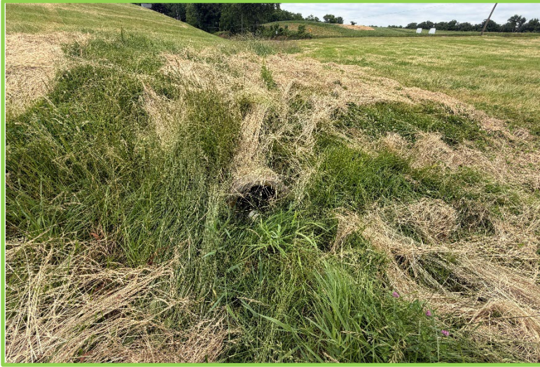
Drainage tile and culvert in ephemeral ditch
