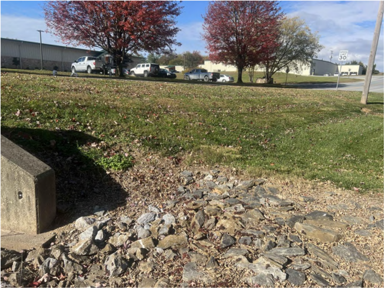
Photograph 13: Culvert at rip-rap apron at the low point of the paper street location on Steel Way Drive (road in background).
